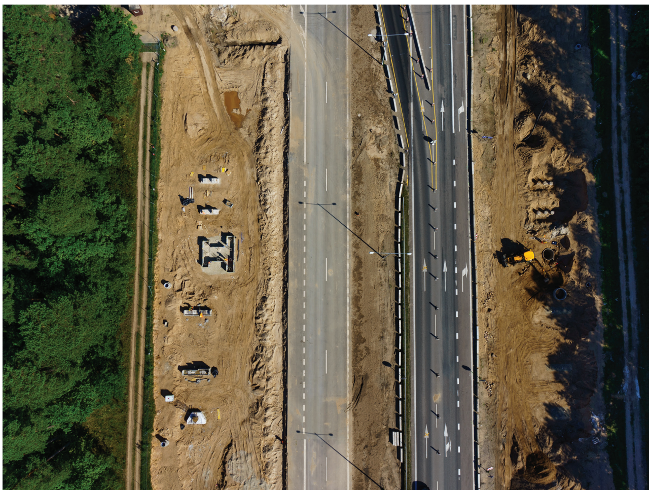
Construction site at Žemaitkiemis junction in Ukmergė district on highway A2 Vilnius–Panevėžys. Construction of support columns for the new pedestrian overpass.
