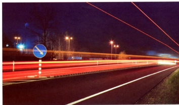
The Main Priority – to Ensure Road Safety By E. Skrodenis
